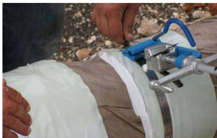
Last wrap of Double-Faced Adhesive with release paper not removed, banding begun.
