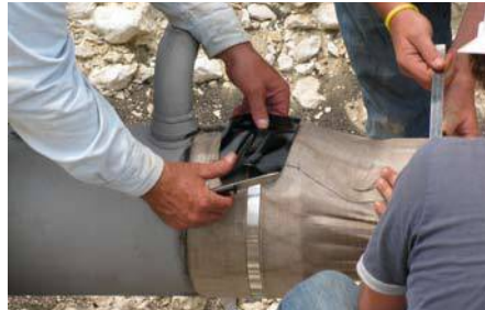
Seal-Wrap banded securely in place and buckles being covered with small squares of Double-Faced Adhesive.
