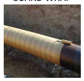
The combination of Innercoat® hot-applied wax and Guard-Wrap $^{\mathsf{TM}}$  is used to prevent corrosion of belowground metal structures.
