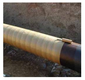
The combination of Innercoat® hot-applied wax and Guard-Wrap<sup>™</sup> is used to prevent corrosion of belowground metal structures.
